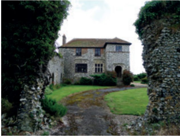
St Radegund's refectory range north wall seen through nave south wall
