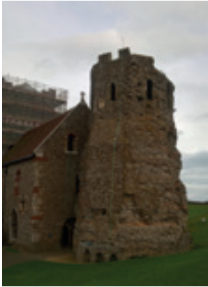
Lighthouse at St Mary in Castro, from the north-west
