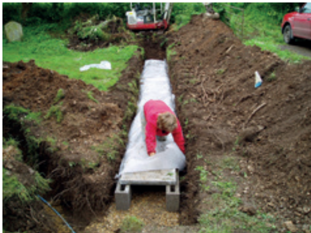
Trench Arch installation at Christ Church Hatherden, Diocese of Winchester
